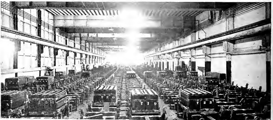
FIG. 1.—BATTERY ROOM OF NEW YORK TRANSPORTATION COMPANY, LIGHTED BY VAPOR LAMPS.
